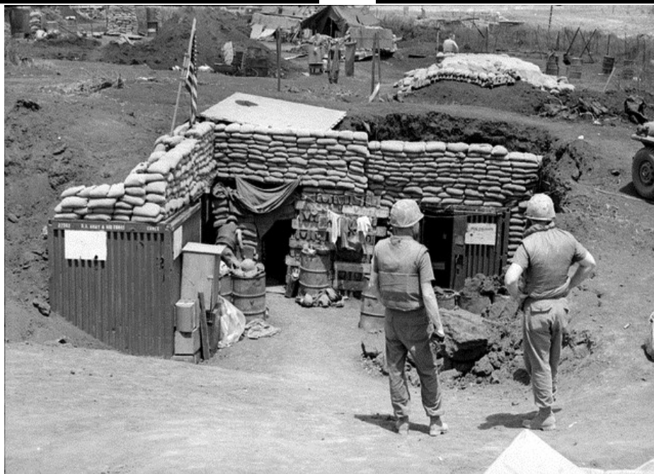
Hilltop in Vietnam, Command post made from Container Express, (CONEX)
